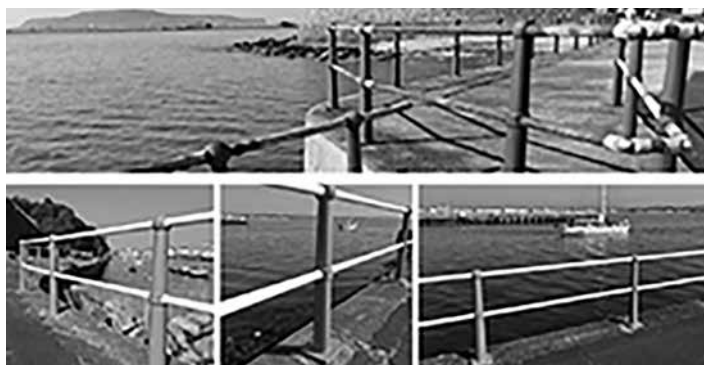
Old and newly painted railings at Weymouth's Stone Pier
