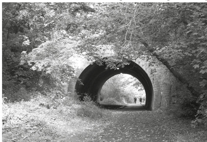
The tunnel on the Rodwell Trail
